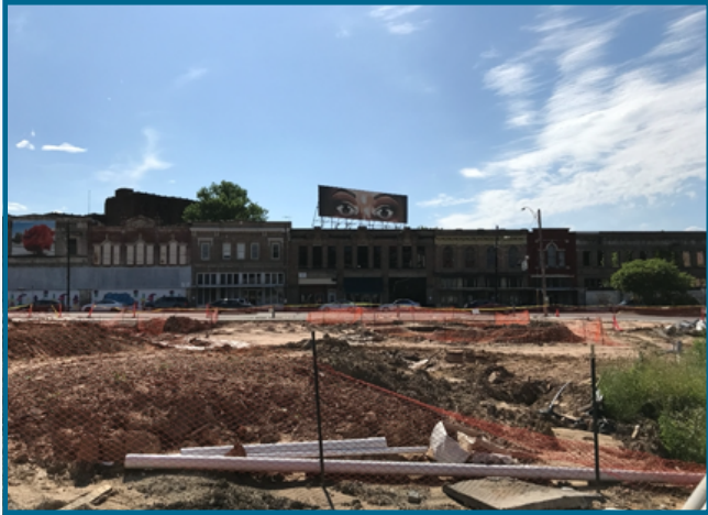
Caddo Common under construction
