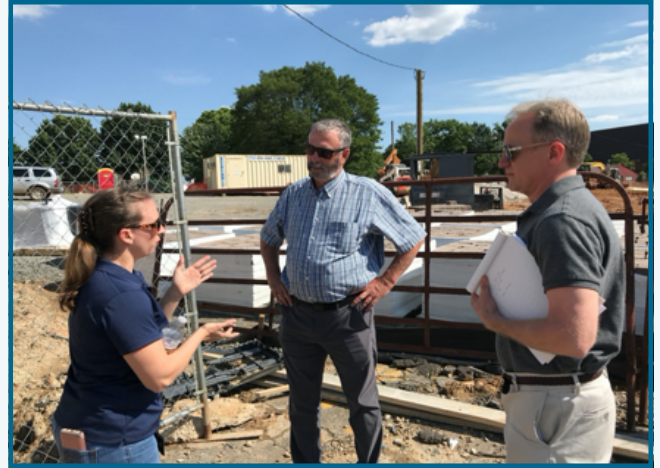
Brandee McCarthy, LDEQ Southwest Regional Office; Duane Wilson, LDEQ, and Wes Wyche, city of Shreveport, survey the construction of the Caddo Common green space.
