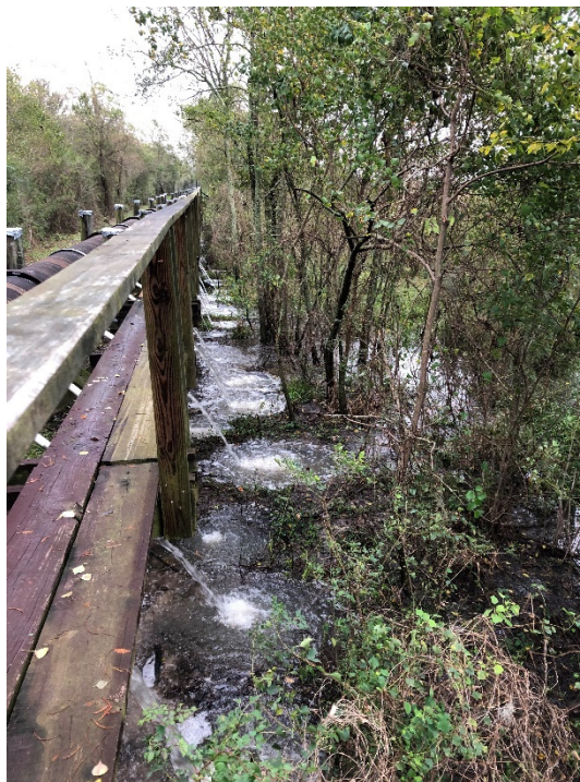
Figure 1 – South Slough Distribution Pipe and Boardwalk
