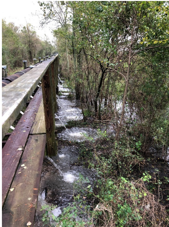
Figure 4.1 – South Slough distribution pipe and boardwalk
