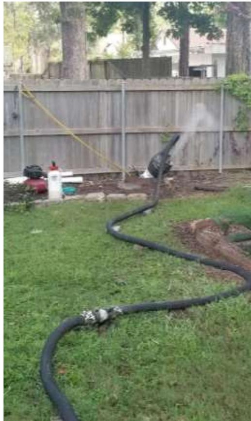
Picture 1: Contractor performing CIPP lining "cooking" process
