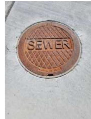
*Picture 1: New Sewer Manhole with new ring & cover along concrete roadway*
