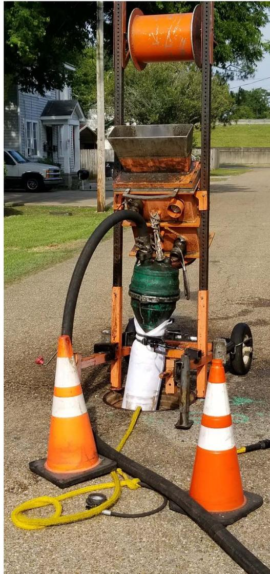
Picture 1: Contractor performing CIPP lining “cooking” process
