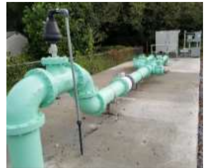
Picture 3: Renovated community lift station
