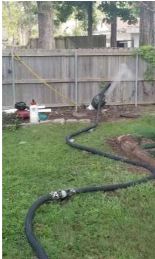
Picture 1: Contractor performing CIPP lining "cooking" process
