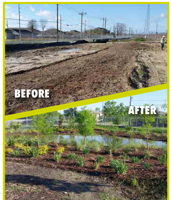
Baton Rouge, LA – South Wastewater Treatment Plant Stormwater Management Completed 2016
