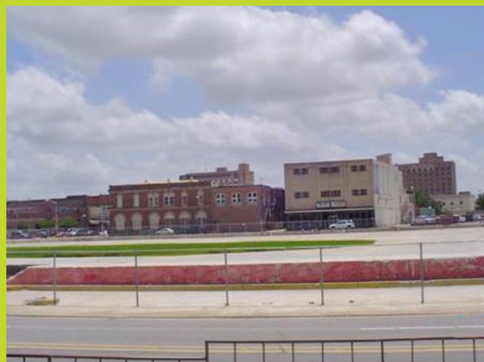
Completed Sears Building in Lake Charles
