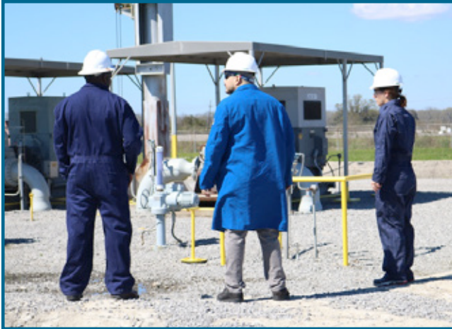
Rogers (r) and Guerrero (middle) meet with a facility representative to conduct a walking tour of the sump units, engines and product tanks to identify any safety or functional areas of concern.
