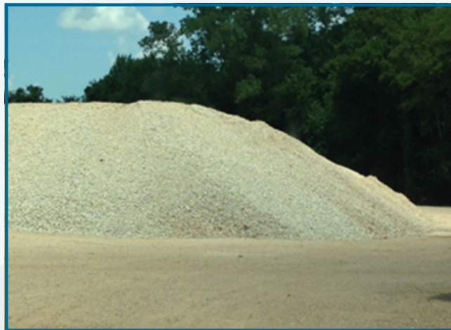
Broken concrete is stacked, crushed, ground down and ultimately repurposed with other material to fill imperfections in the runway.
