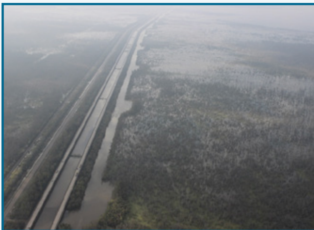
Flooding alongside a stretch of Interstate 55 in Tangipahoa Parish north of Lake Maurepas.
