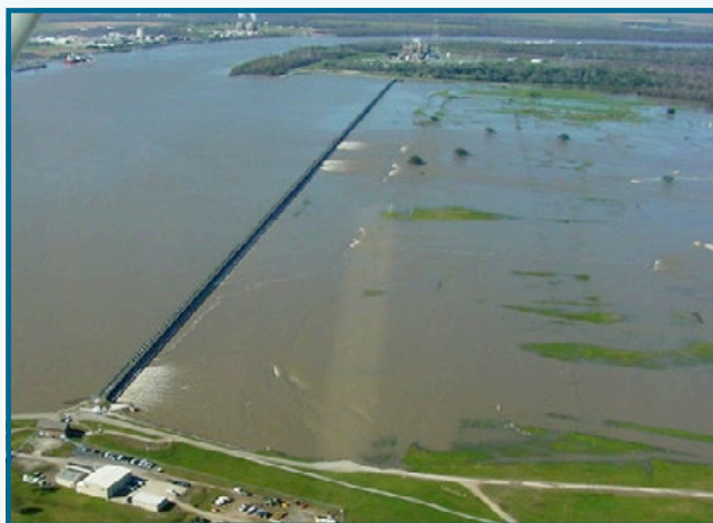
Bonnet Carré Spillway opening shown from an overflight conducted by DEQ on Jan. 11. The flow rate at that time was 299,200 gallons per second discharging through 38 of the Spillway's 350 bays.
