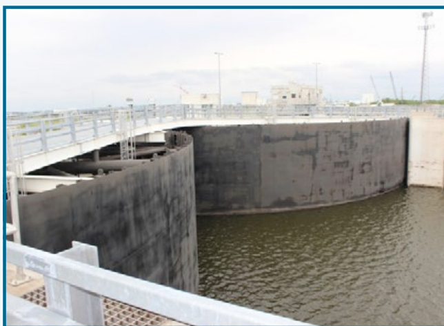
The fully closed front side of the sector gate of the Gulf Intracoastal Waterway in eastern New Orleans.
