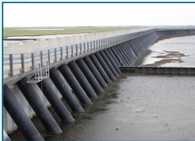
The storm surge barrier along the Inner Harbor Navigation Canal in eastern New Orleans is comprised of a 1.8 mile wall with three gating systems.
