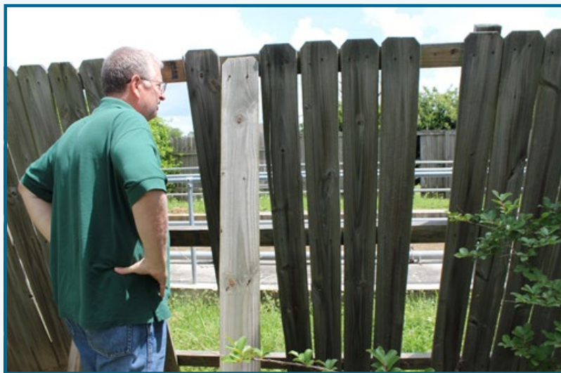
Adequate fencing is needed around wastewater treatment units, as DEQ Environmental Scientist Don Weinell conducts a site inspection in Ascension Parish
