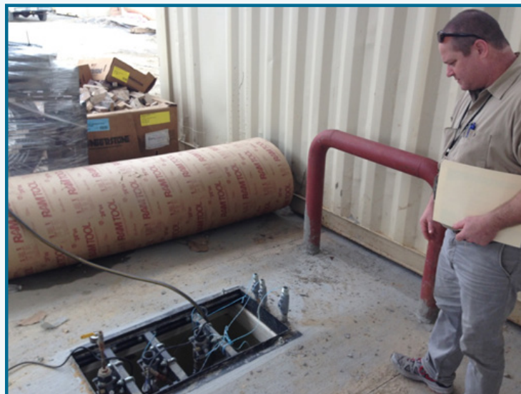
Environmental Scientist Laurence Carter checks a gas station's fuel dispenser site for proper drainage and safety protocols.
