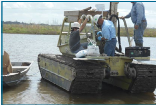
During the sampling process, contractors use a drill that has a bentonite seal between outer drill case and the inner drill hole. This keeps pond water from entering the aquifer or compromising the sample.
