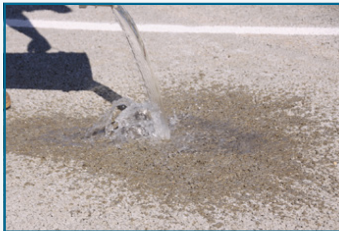
Project engineer Henry Shuler pours five gallons of water onto the pervious concrete parking lot adjacent to the Winn Parish Courthouse in Winnfield. The water soaked in almost instantaneously.
