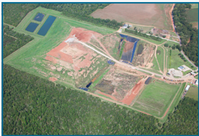
Aerial View of the St. Landry Parish Landfill
