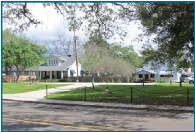
The Timeless Treasures site after completion at 121 Bridge Street in New Iberia.
