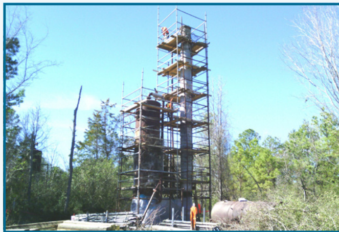
Removal work in progress at the Ida Refinery cleanup in Ida.
