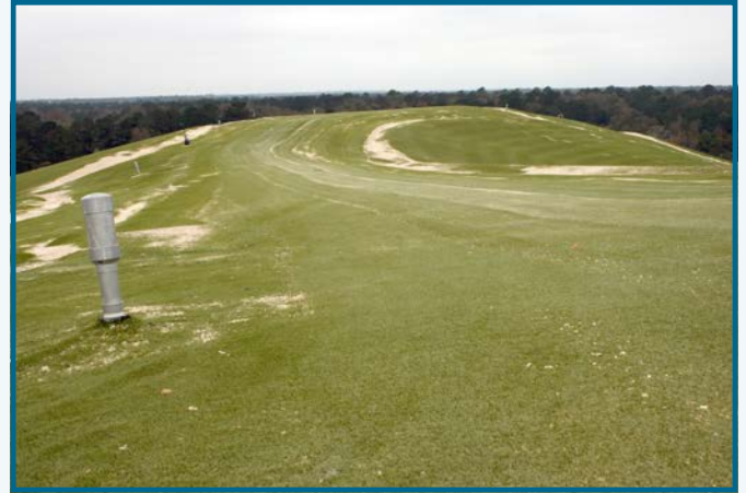
Gas collection wells dot the artificial turf covering Cell 10 at the Tangipahoa Parish Solid Waste Facility near Independence.
