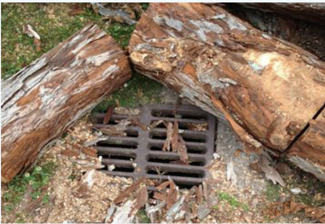
Tree debris obstructing storm drains poses health, safety and environmental hazards
