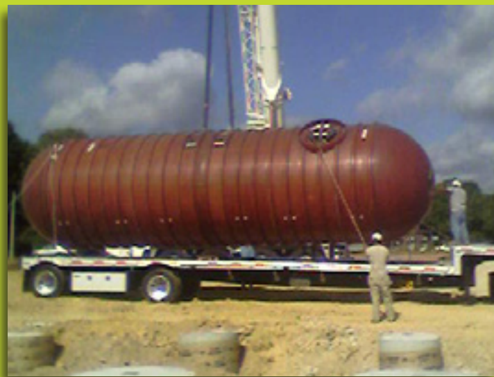
Workers install Underground Storage Tank
