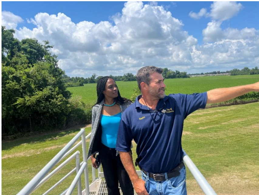
Secretary Giacometto surveys the city's wastewater facilities with Carencro Water Supervisor Buster Broussard.
