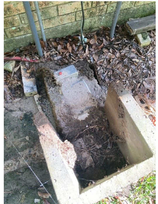
Figure 3 – Overflow from waste tank needing to be pumped out due to aerator not functioning
