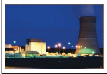
A Nuclear power plant uses steam to generate electricity. Steam, created by heating water though energy produced by a nuclear reaction, drive turbine blades to spin. This rotational energy is then converted to electrical energy by a generator.
