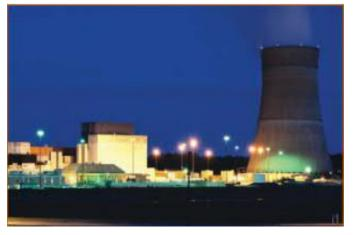
A Nuclear power plant uses steam to generate electricity. Steam, created by heating water though energy produced by a nuclear reaction, drive turbine blades to spin. This rotational energy is then converted to electrical energy by a generator.
