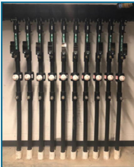
The geothermal system is continually monitored to ensure that the system is working properly.
