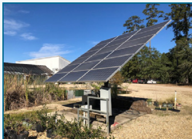
Solar panels at the Sustainability Center capture energy that helps to power the Center
