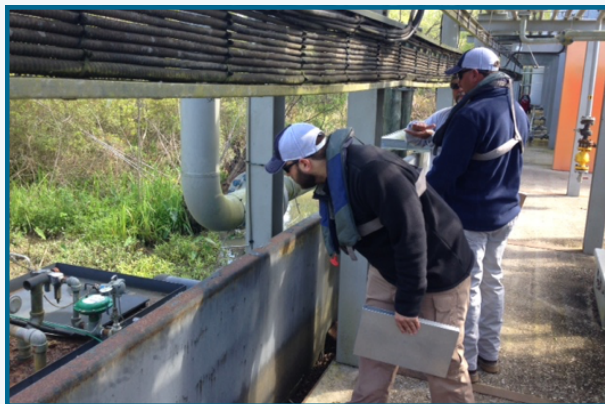
LDEQ Environmental Scientists Andrew Kimmel (left) and Carrick Boffy accompany an oil facility operator on a tour as they inspect the platform's water/oil separation equipment in St. Mary Parish.
