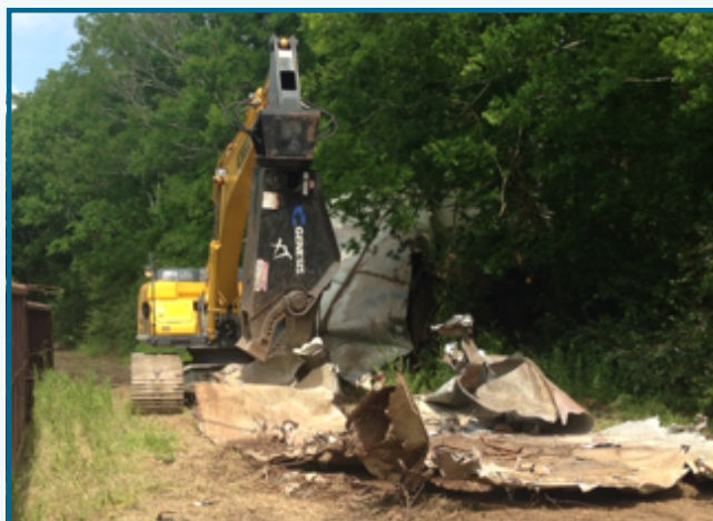
During the tank removal and cut-up process, special shears were affixed to a hydraulic excavator, which cut and flattened the steel for ease of disposal.
