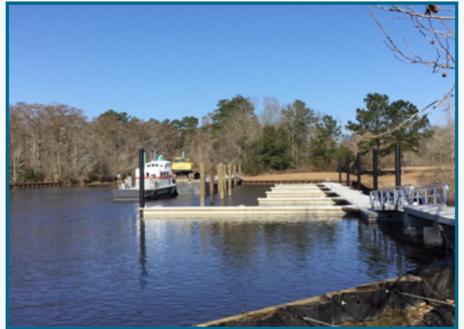
The addition of a dock is part of the revitalization effort at Bayou Bonfouca. Photo courtesy of EPA.
