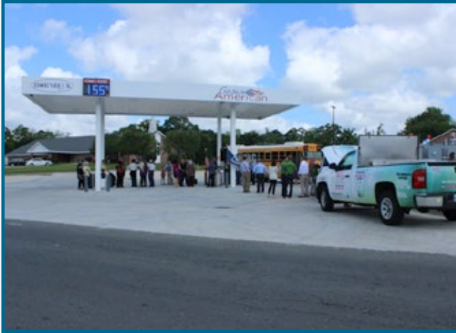
Hornbeck's CNG fueling station looks like a typical gasoline fueling station.
