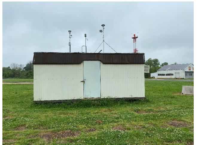
Shreveport Airport AQS 22-015-0008
