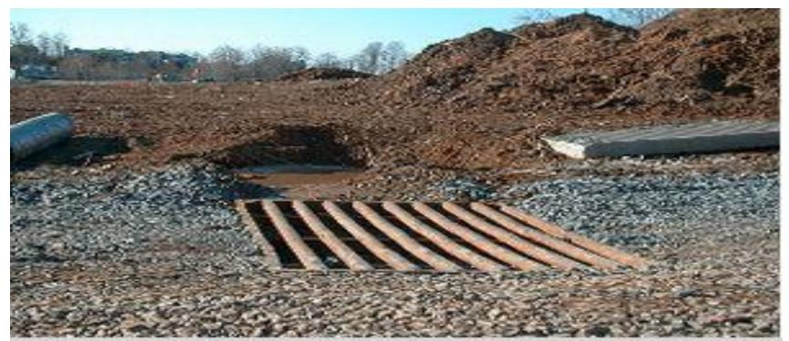
Stabilized construction entrances allow dirt to be removed from tire treads and collected as trucks leave construction sites
