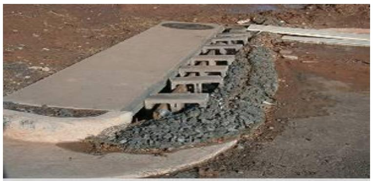
Coarse gravel and cinder blocks are often used to keep sediment and other pollutants out of storm drains
