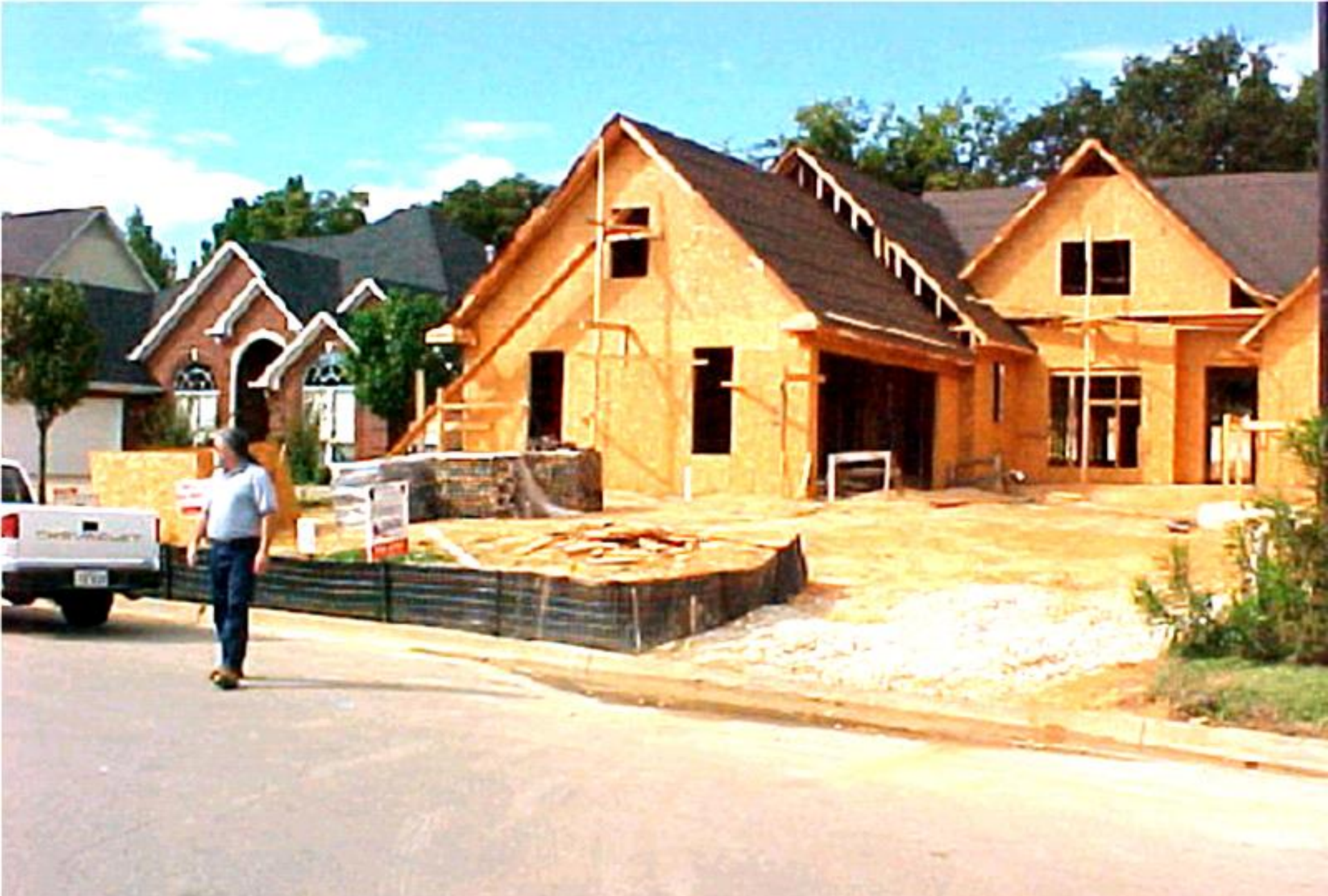
Properly installed and maintained silt fence.
