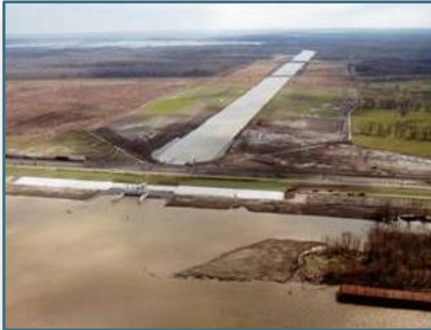
Figure 20. Example of an existing diversion Davis Pond Freshwater Diversion connecting the Mississippi River (foreground) with coastal wetlands (background).
