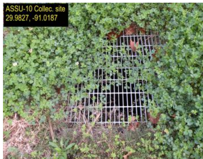
Sample collection culvert on the Bayou side at LA Hwy 1.
