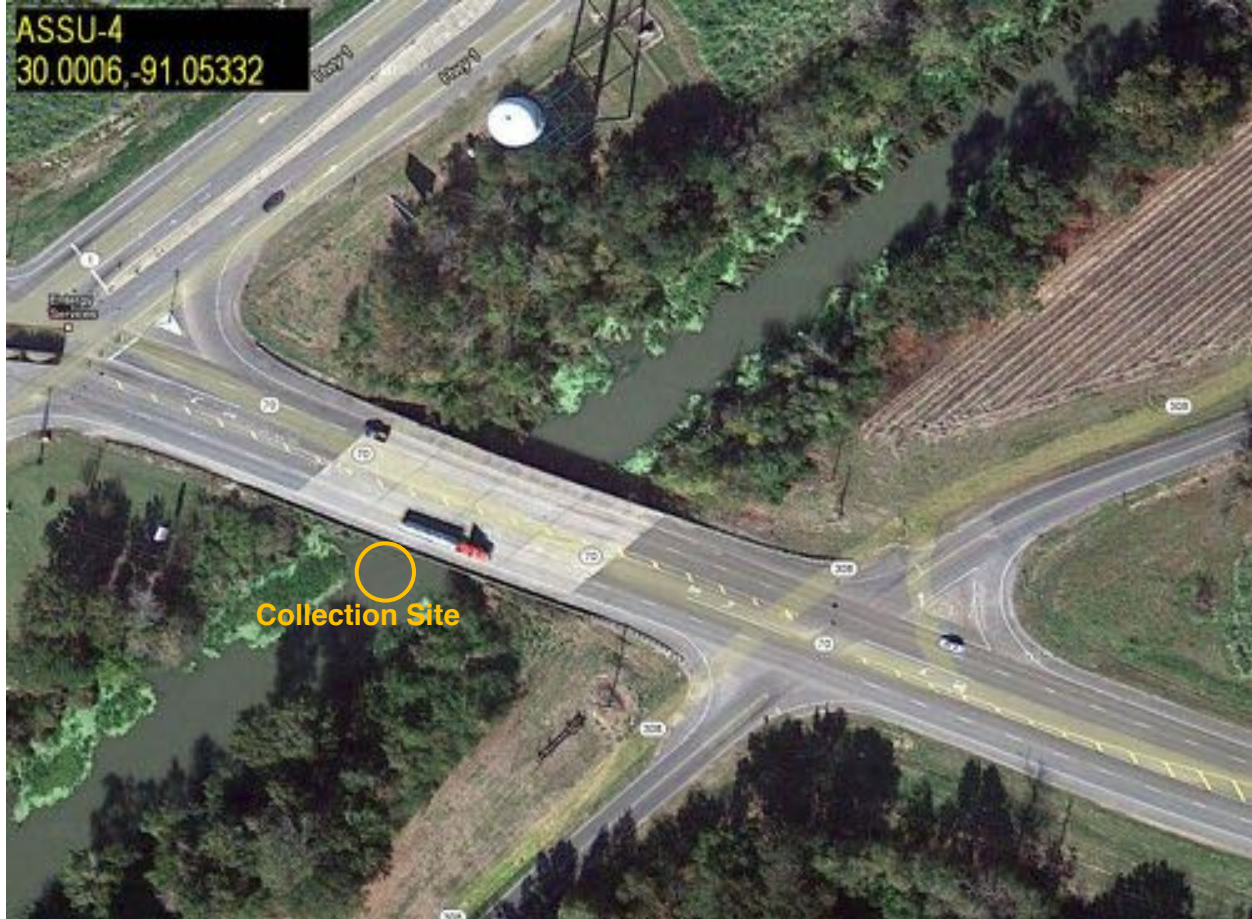
The ASSU-4 Spur 70 bridge travels east across LA Hwy 308 to the Sunshine Bridge and west across LA Hwy 1 to Pierre Part.
