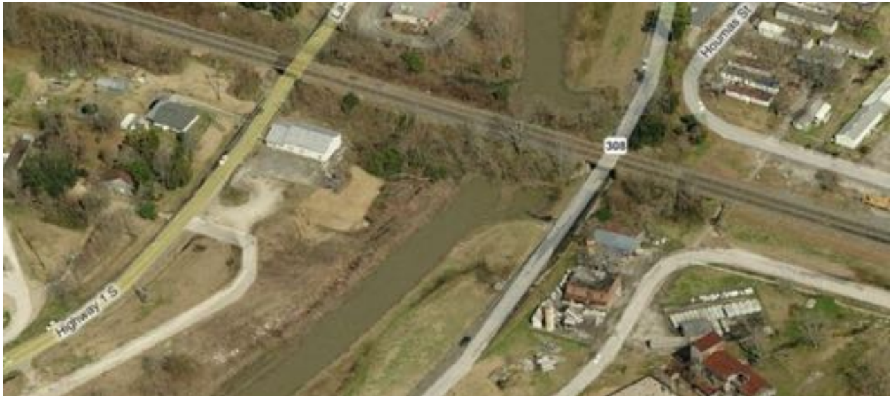
Railroad earthen dam crossing over Bayou Lafourche in Donaldsonville. Congestion with trees and brush clearly is blocking the flow from the river.
