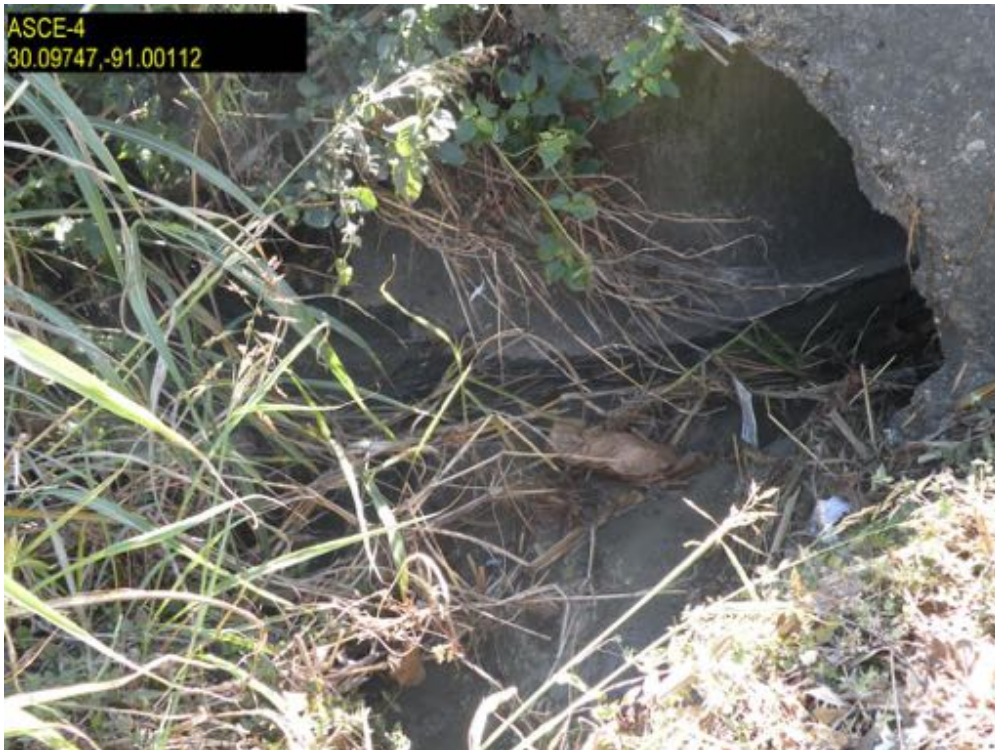
ASCE-4 Collection Culvert at Popeyes on Bayouside in Donaldsonville. Drains into Bayou Lafourche behind Popeyes.
