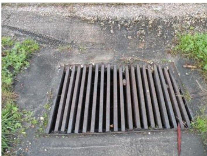
Culvert in Church parking lot on LA Hwy 1
