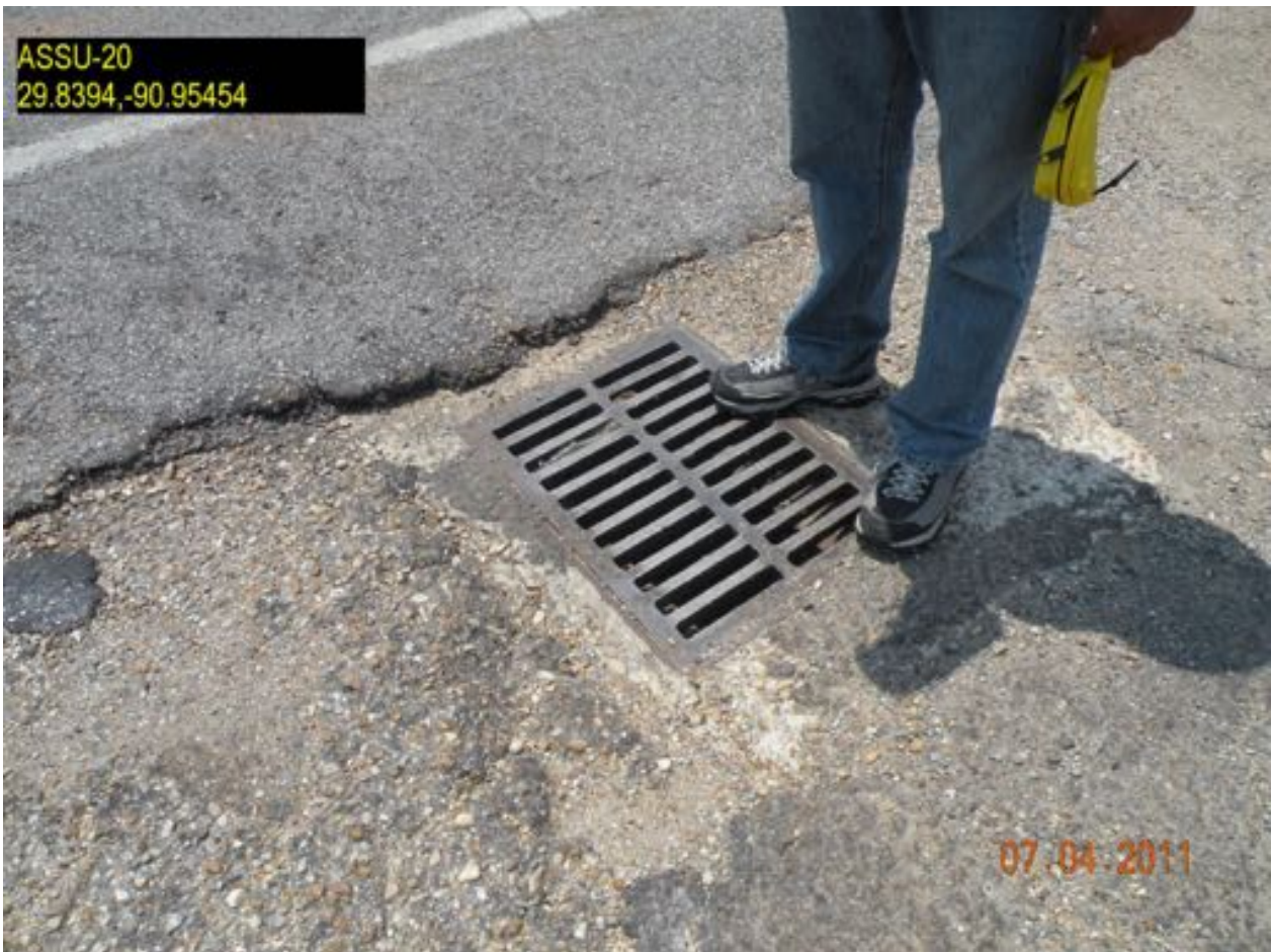
Dr. Balji standing at ASSU-20 storm drain culvert to get GPS coordinates of this collection site. ASSU-20 is a HOT SPOT . This culvert drains towards the Bayou under LA 1 into another culvert and directly into the Bayou.
