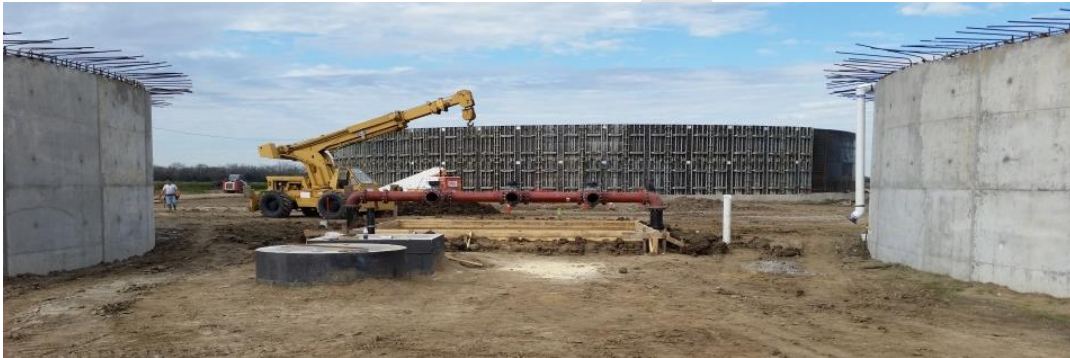
Picture 4: New Regional Wastewater Treatment Plant
