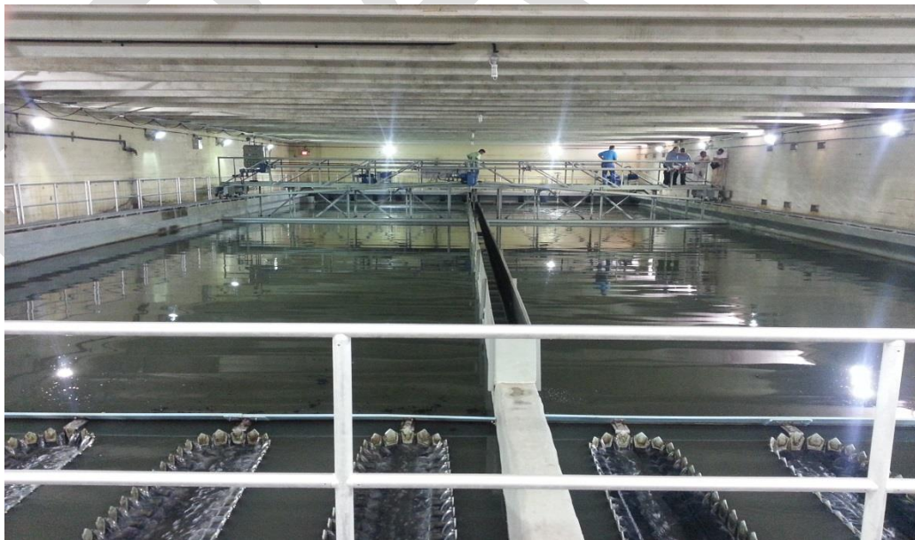
Picture 3: Wastewater Treatment plant rehabilitation project (consisting of clarifier traveling bridge replacement and concrete repair / coating)
