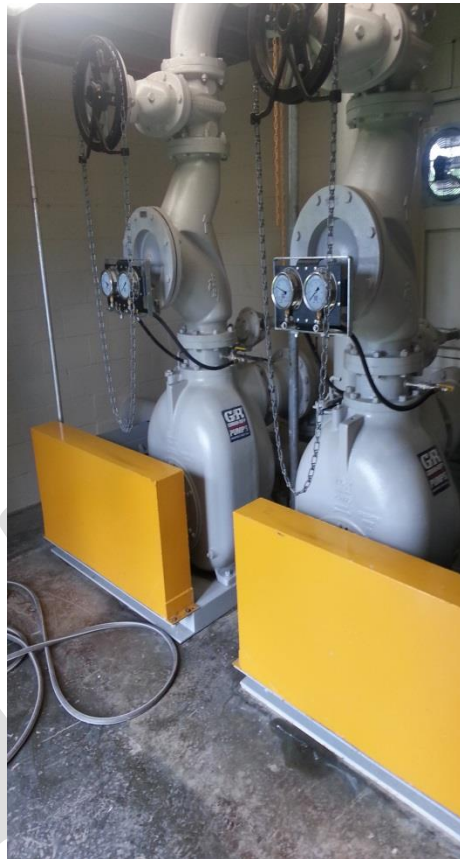
Picture 1: New pumps, piping, valves, and appurtenances in an existing pump station rehab project.
