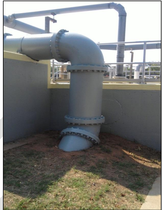
Picture 2: Wastewater Treatment Plant Headworks rehabilitation project
