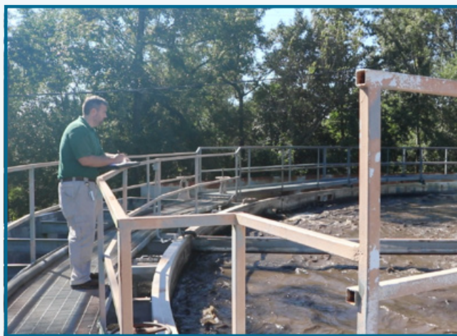
LDEQ engineer William Barlett examines a POTW for CWSRF requirements.
