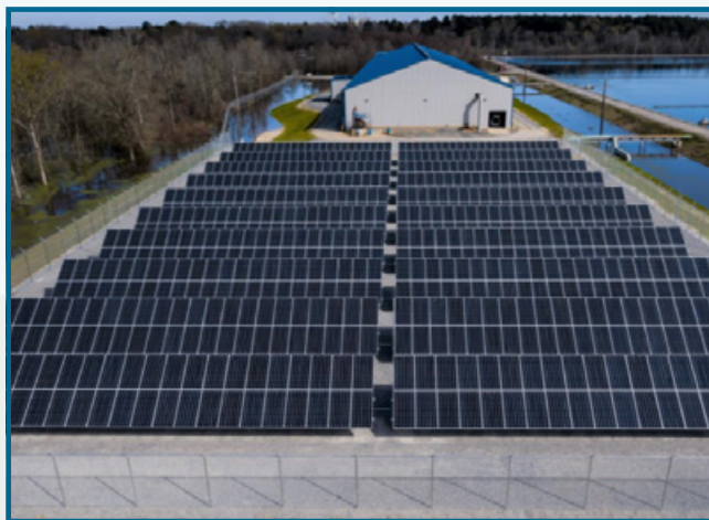
2017 Award Recipient: City of West Monroe – Wastewater Treatment Plant Solar Farm
