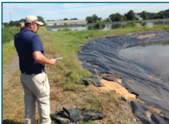
During a walking tour of the site, LDEQ Environmental Scientist Staff Jeremy Moore will observe the conditions of the aeration ponds, identifying any imperfections in the plastic liner (such as the tear seen here), the existence of any strong odors, if high vegetation or obstructions are affecting the ponds, and whether solids are in the water. Inspectors also check to see that the aerators are functioning properly.
