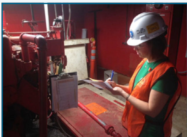
Kelly McDermott examines the facility's fire pump and diesel engine unit during an inspection.
