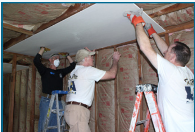
LDEQ's Bob Bailey, center, helps install Sheetrock on the ceiling of the home of Lorenzo and Janice Angel.
