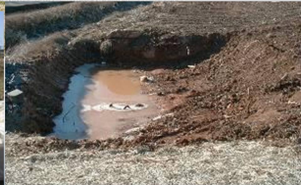
Sediment traps are used to collect sediment-laden runoff from disturbed areas on construction sites
