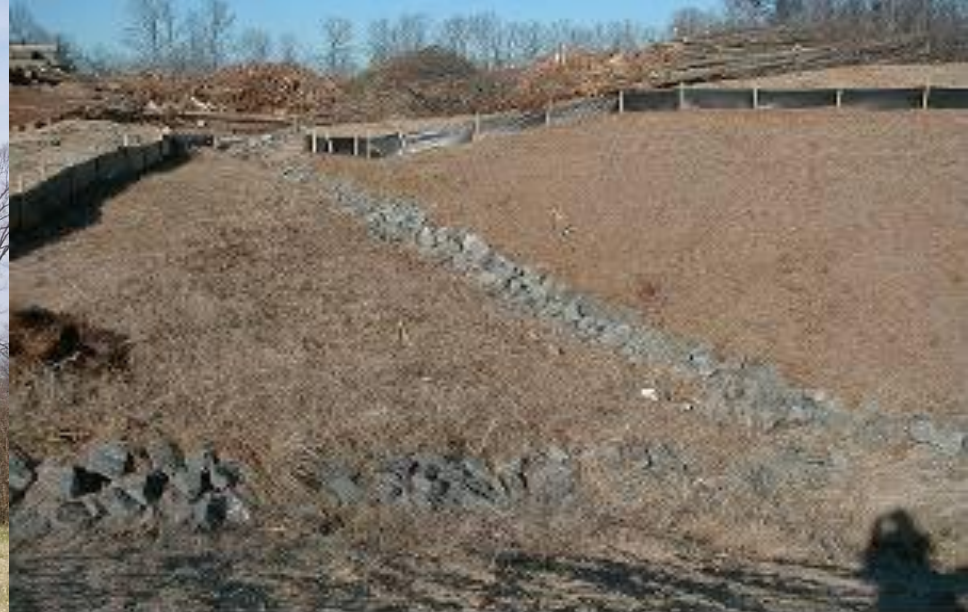
Riprap can be used to stabilize drainageways and outlets to prevent erosion
