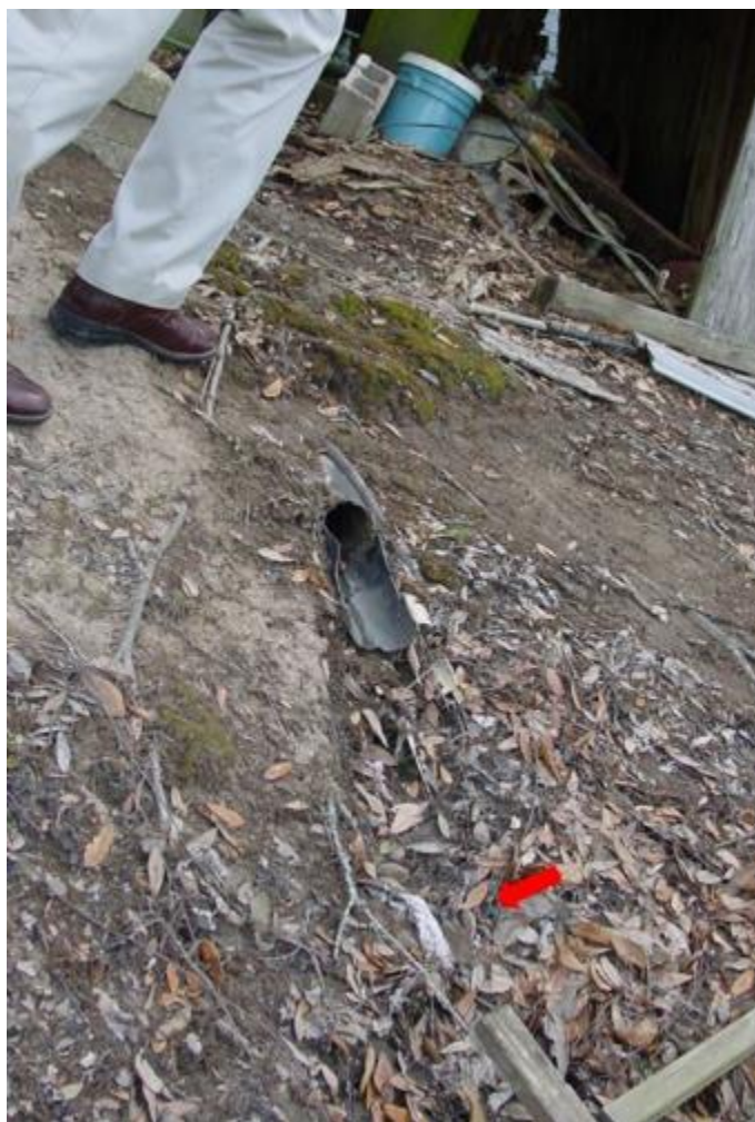
Figure 16. Raw sewage with toilet paper discharge from home onto bank of waterbody
