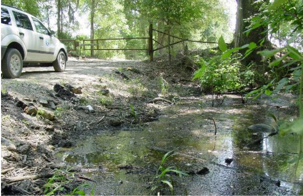
Figure 12. One of many driveways acting as dams on Bayou Maringouin south of I-10, completely blocking the flow of water.
