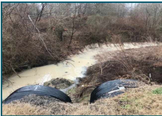
Figure 4. Site 4688 [Unnamed tributary at La Hwy 576] - Canal Dredging
