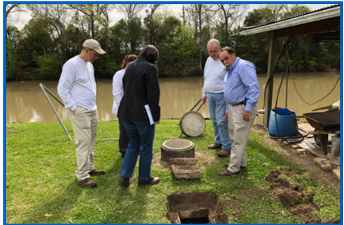
Rusty Reeves, LRWA Deputy Director, Training Specialist (right), explains the operation of an onsite wastewater treatment system in Thibodaux. The training was part of a home owner's wastewater treatment system maintenance class conducted by LRWA, LDEQ, and LDH.
