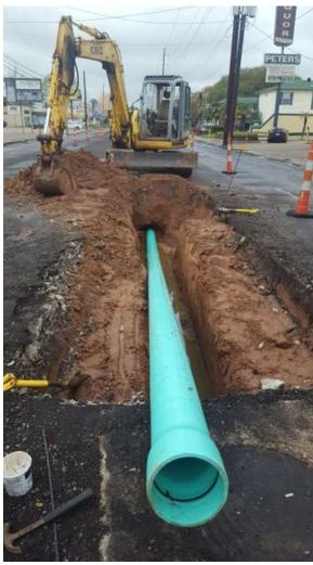
Picture 2: Collection system Rehabilitation – Pipe Removal and Replacement
