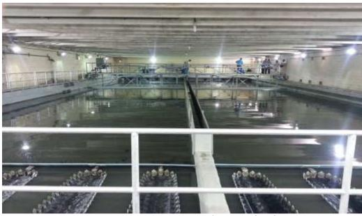
Picture 3: Wastewater Treatment plant rehabilitation project (consisting of clarifier traveling bridge replacement and concrete repair / coating)
