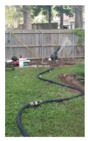
Picture 1: Contractor performing CIPP lining "cooking" process
