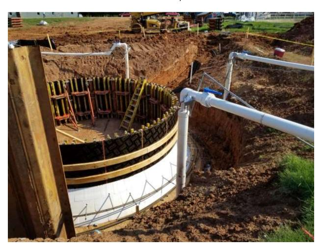
Picture 4: Contractor using a well point system when installing an influent wet well caisson at a WWTP
